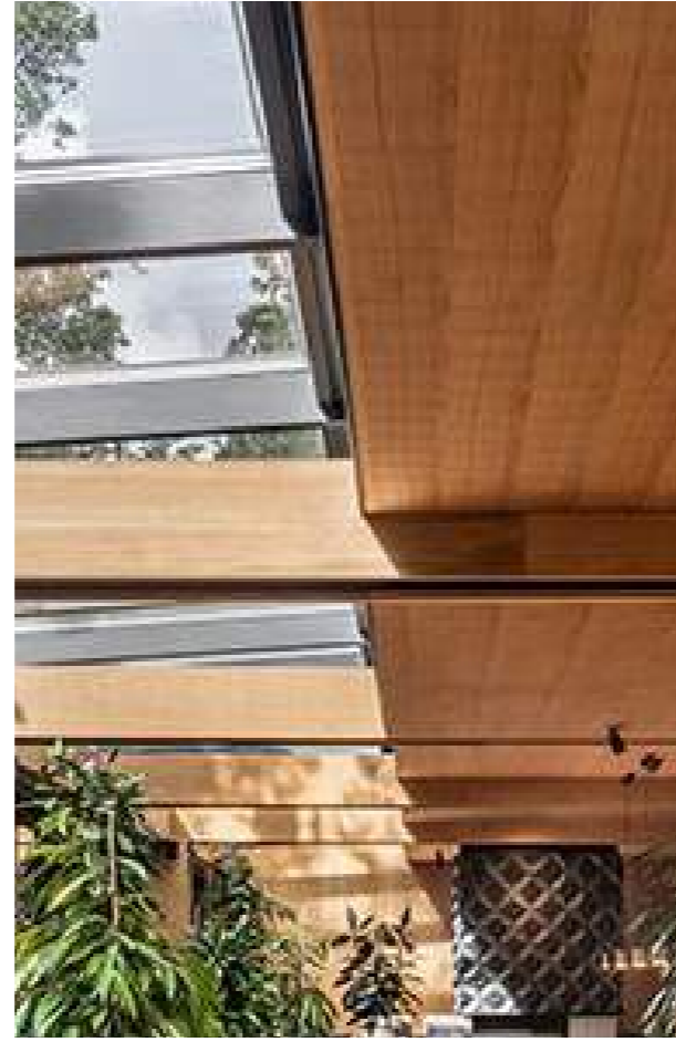
Timber Lined Ceiling
